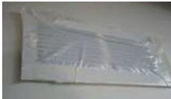
Figure 10: Seal all supply and return registers with Grill Mask
