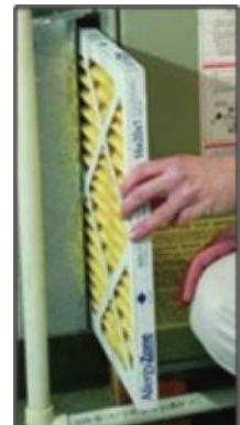
Figure 11: Remove all air filters
