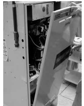
Figure 20: Preparing to connect to ducts via air handler
