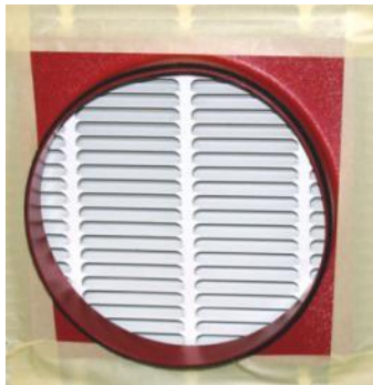
Figure 19: Flange taped onto a return register before attaching the Flex Duct
