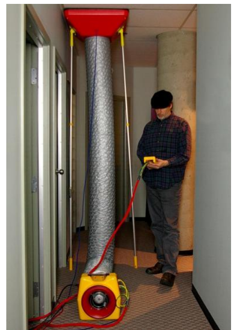
Figure 28: Measuring air flow with a Powered Flow Hood
