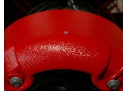
Figure 17: Pressure sensor on the fan motor casing.
