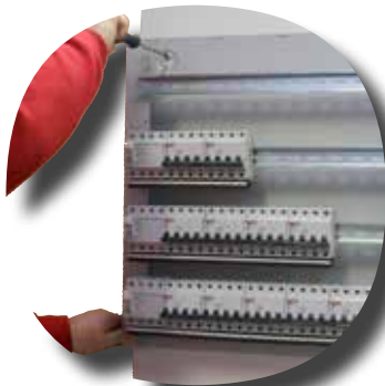
The rear plate is fitted on the wall.
