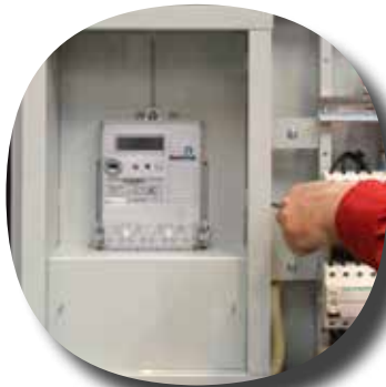
Meter insert mounted - accessory.
