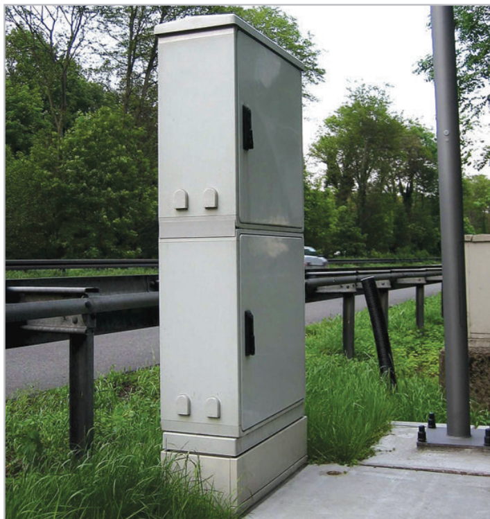
Cabinet can be provided with door on the front and at the rear: easy access, two different individual compartments.
